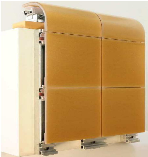
Kuwait National Museum Treasury – model of internal wall cladding system developed by 3form for Varia Ecoresin, design Studio A London
